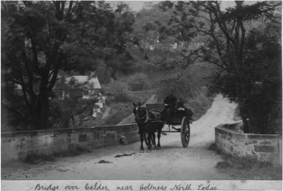
FIGURE 4. Bridge approach to Coltness House, former estate of Coltness
