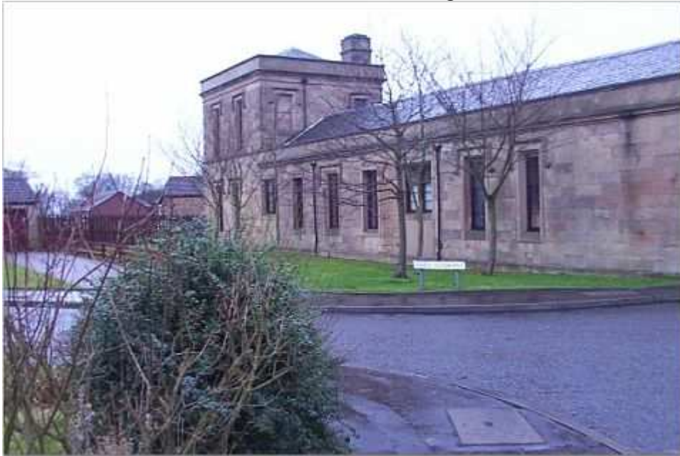
FIGURE 7. Remains of Coltness House outbuildings II, 2002.
