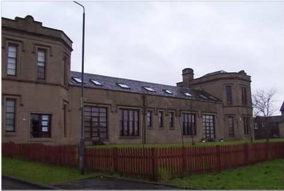
FIGURE 6. Remains of the Coltness Outbuildings I, 2002
